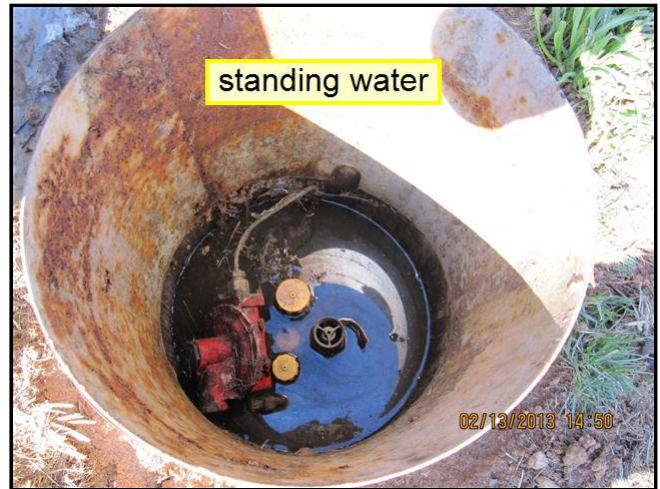
6.4 Picture 2 propane tank valves
